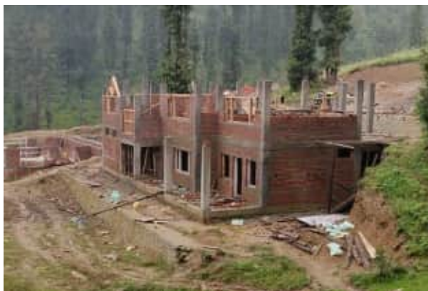
Interpretation centre (in construction stage)
