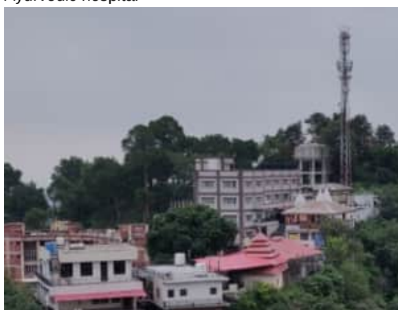
Water tank & mobile tower
