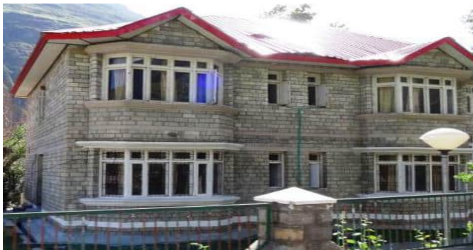
Exhibit 10.166: PWD Guest house, Sissu
