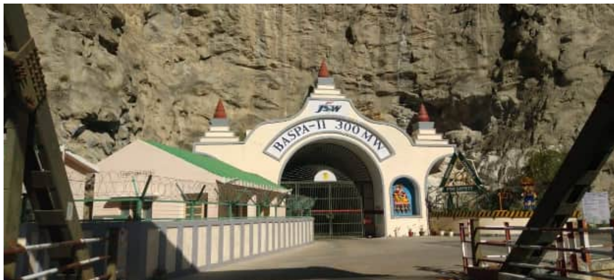
Exhibit 10.242: Baspa Stage II Project is the first Independent Power Producer (IPP) project after the Government of India
