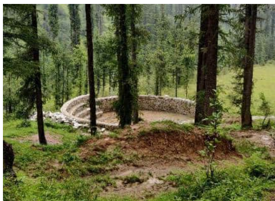
Amphitheatre (in construction stage)
