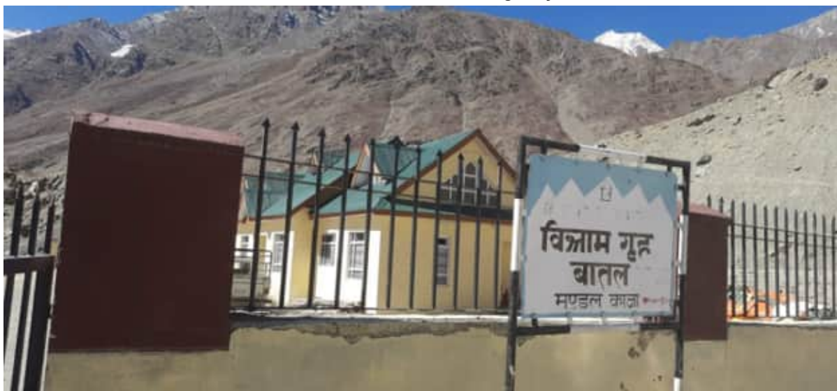
Exhibit 10.195: PWD Guest house Batal, on the Sissu – Kaza highway
