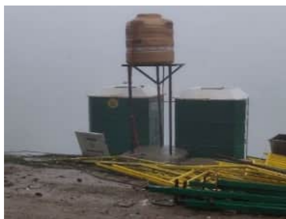
Exhibit 10.83: Public toilet at the entry point to Shikari Devi Temple area
