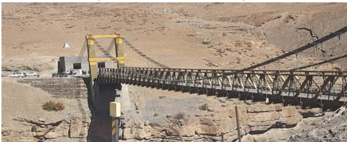
Exhibit 10.181: Chicham Bridge on Samba Lamba Nallah, Cheecham village, Cheecham Kibber road
