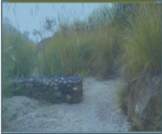
Toe wall has been exposed, H is too small for given length
