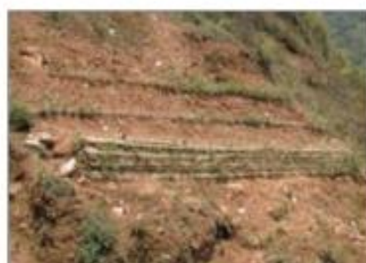
Bamboo Crib Wall Construction
