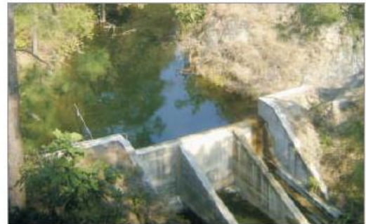
Masonry Drop Structures (1.5-2.0 m height for Silt & Runoff Control)
