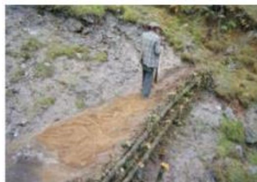
Bamboo Crib Wall Construction
