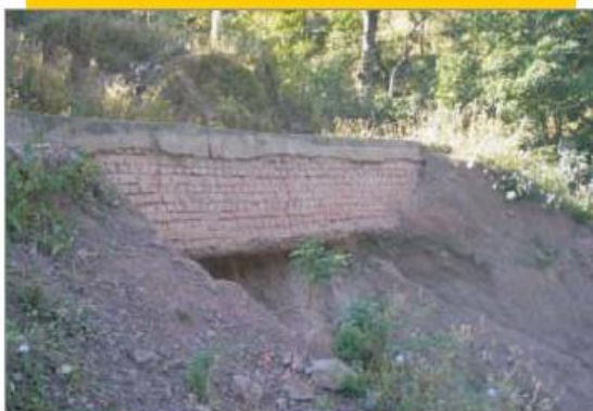
Defective Foundation Work
