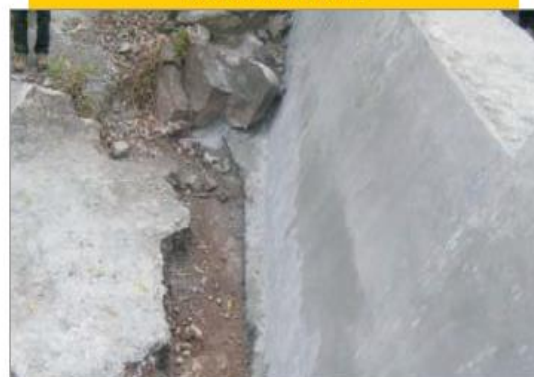
Defective Foundation Work
