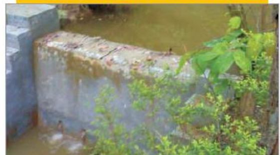
Masonry Drop Structures (1.5-2.0 m height for Silt & Runoff Control)
